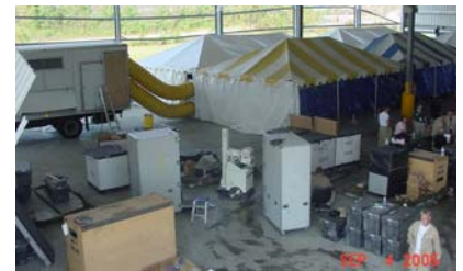
DPMU with air conditioning completed 9-4
