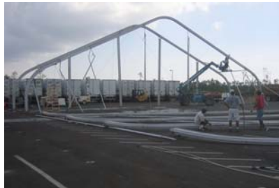
DPMU tent being erected
